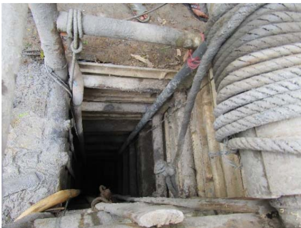
Gambar 7. Lubang Masuk Vertikal (Shaft)
